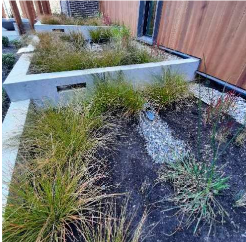
1. Terraced rain gardens along building.
